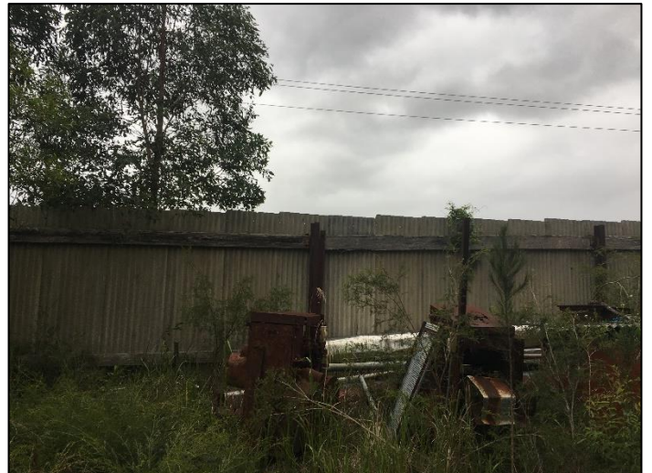
Plate 18: ACM along the eastern boundary of the site.
