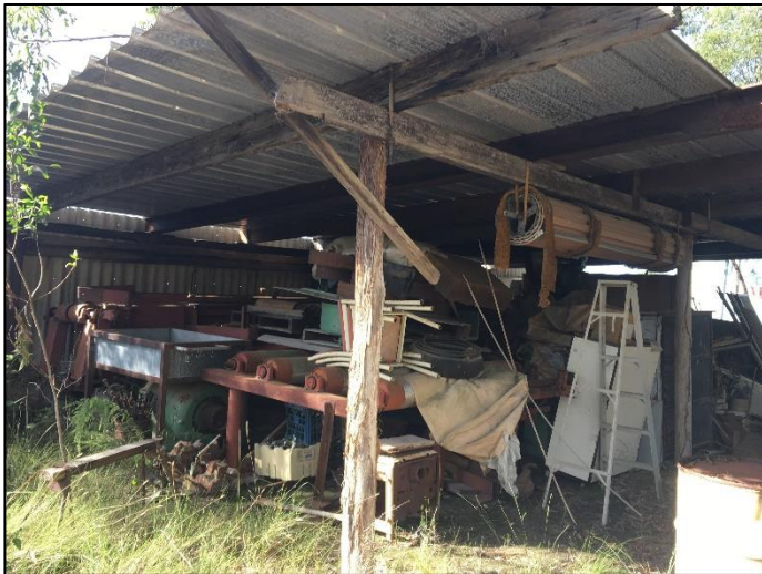
Plate 21: Maintenance shed on the central eastern boundary of site looking south east.
