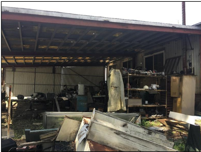
Plate 15: Metal clad shed north of the dwellings.
